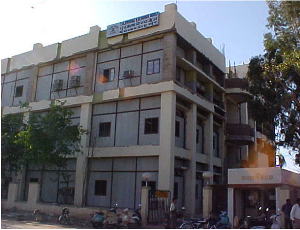
Figure 16-4. The large panel burnt-clay brick masonry infills in cement mortar, sustained partial collapse at the upper story of the three-story telephone exchange building in Bhuj. The infills of the entire building, including those at the lower stories, were replaced with lightweight foam concrete panels sandwiched between asbestos sheets. These panels were secured to the frame with thin steel straps.
