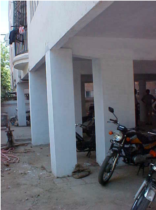
Figure 16-9. RC frame buildings with open ground stories usually have overhanging beams along the perimeter in the ground storey. Many of these cantilevers sustained shear cracks during the earthquake. In this building, masonry columns were constructed under the tips of these beams as a retrofit measure.
