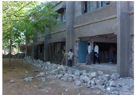
Figure 16-3. Large block sandstone masonry infills in cement mortar at a two-story school building in Ahmedabad were completely replaced with burnt-clay brick masonry infills in cement mortar.
