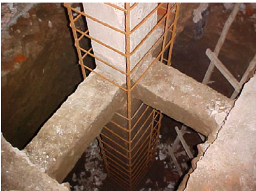
Figure 16-13. Instances where column jacketing was started at the footing level were few. Even in these cases, the column reinforcement may not have been anchored into the footing and even the footing may not have been enhanced.
