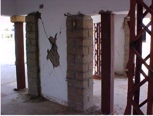
Figure 16-7. RC columns of the three-story residential RC frame building in Gandhidham are adjoined with brick masonry columns from the floor level to the beam soffit. The beam is propped at intermediate locations with hot-rolled steel I-sections.
