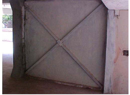
Figure 16-8. Steel braces are employed in limited cases to strengthen the open ground story panels. This picture shows bracing employed in addition to the infilling with burnt-clay brick masonry infills and jamming of steel sections at the outer faces, in a residential building. The bracing member used is a steel hollow box-section of 100 size with 8 mm plate thickness.
