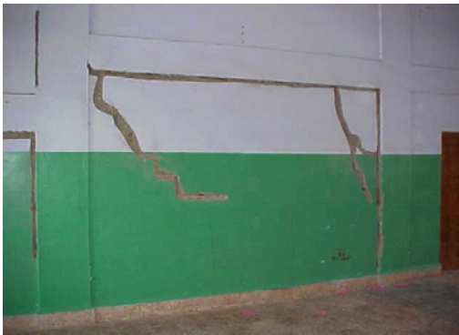
Figure 16-2. Numerous buildings in the affected area sustained only frame-infill separation. In most of these cases, the separations were cleaned and filled with rich cement mortar. The above picture shows the repair done at a school building in Gandhidham.
