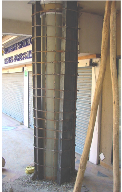
Figure 16-6. The circular RC column in the ground story of an 11-story (including a basement story) commercial building in Ahmedabad is jacketed with hot-rolled I-sections with ties to hold it adjoining the concrete column. There are no connections between the RC column and the steel I-section.
