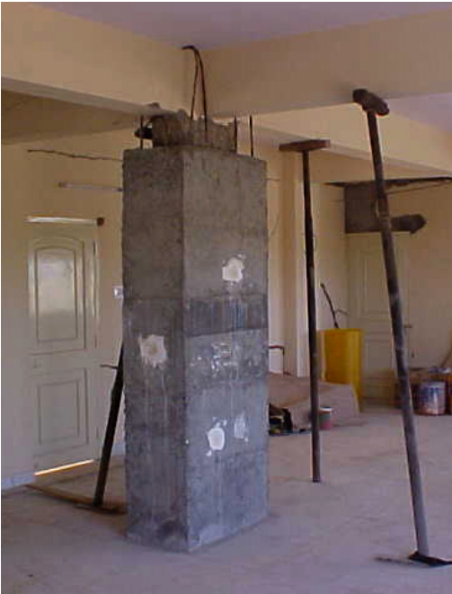
Figure 16-5. Jacketing of a rectangular column of the ground story of a seven-story old age home in Gandhidham, was performed from the floor level to a level well below the beams at the top of that column. The column bars are seen curtailed by the side of the beam.
