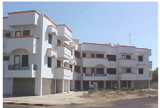
Figure 16-10. In this RC frame building with open ground story masonry infills were provided in select panels of the ground story without hampering parking in the open ground story.
