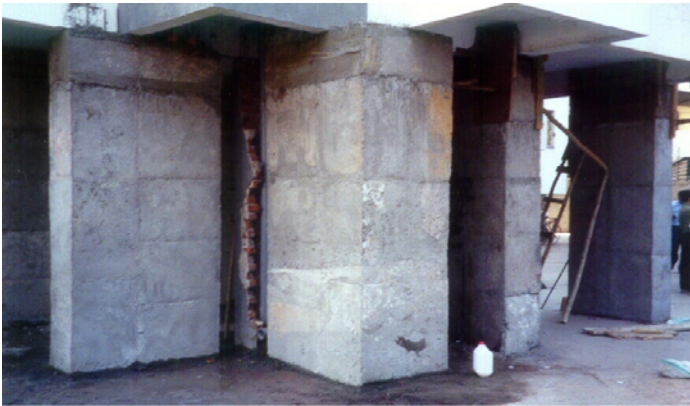
Figure 16-12. The open ground stories in RC frame buildings were intended to provide parking in the ground story. In some cases, this function was hampered after jacketing, because the size of the jacketed columns did not leave much space for movement, particularly for cars.
